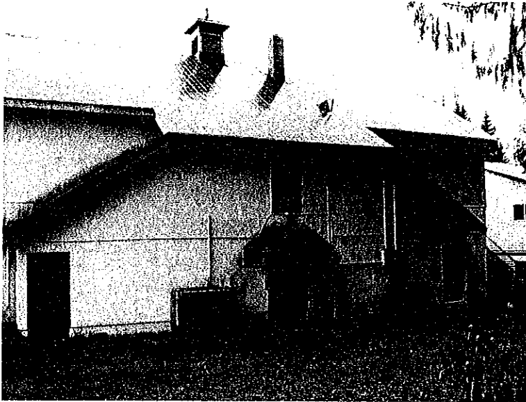
Figure 1: Rear of building.
