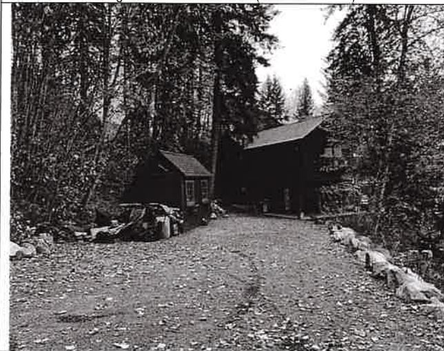
Photo 3: Shed and house on property bench (east view)
