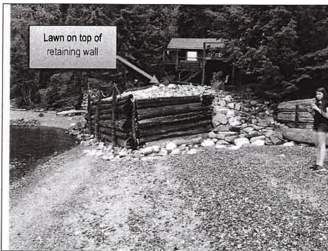
Photo 1: Retaining wall conditions in 2015 (east view)
