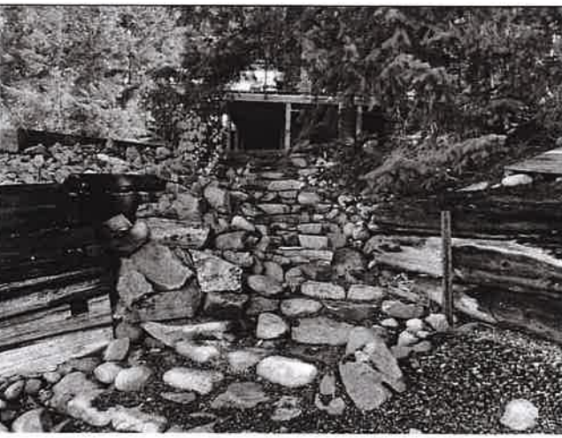
Photo 6: Rock stairway to access top of retaining wall (east view)
