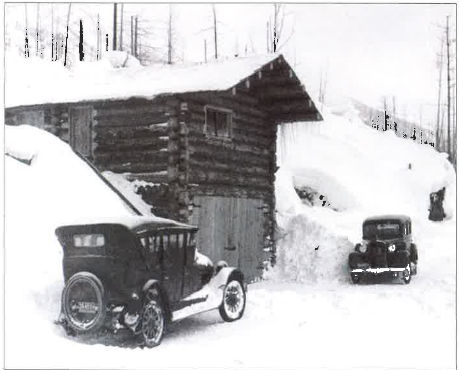
Caterpillar house south of Summit Lake (1935) was built to house highway clearing equipment on ground level. Living quarters for the operator and maintenance man were above. In bad weather they could work out of here in both directions, north to Nakusp and south to Rosebery. — SSHS ARCHIVE PHOTO A006-008-039
